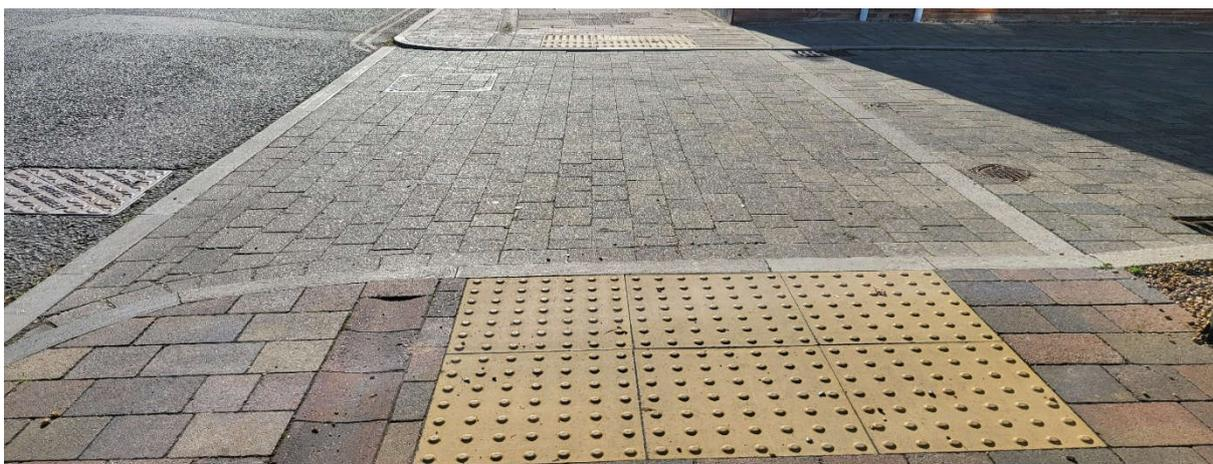
Figure 16 – Example of an accessible junction for all NMUs
