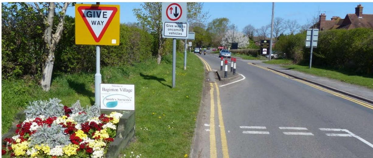
Figure 25 – Example of a priority give-way system
