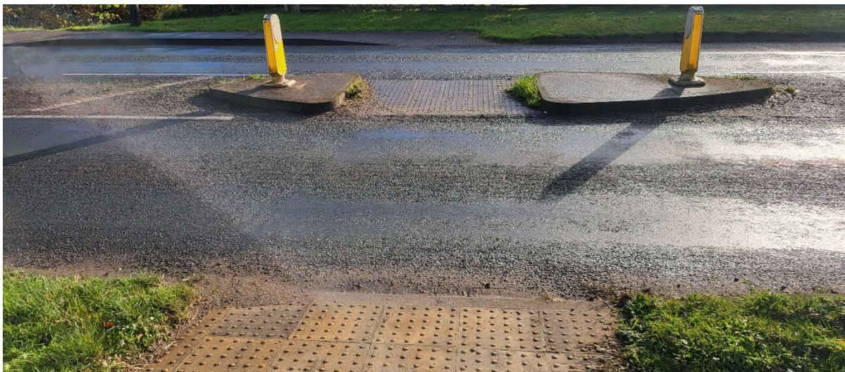
Figure 21 – Example of uncontrolled crossing
