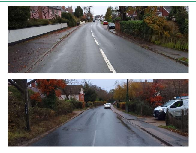
In removing the centre line marking it can reduce the drivers confidence to travel at excessive speed by ensuring that there is no defined area to travel on the road. This lack of confidence in the position you undertake when travelling means that the driver at times will decrease speed because of potential conflict on the carriageway.
