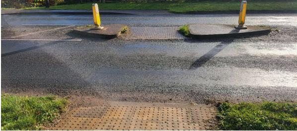
Figure 21 – Example of uncontrolled crossing
