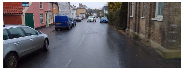
There are also examples of locations within Stradbroke where there is a footway provision but insufficient in width to be accessible to all users. An example of this is along New Street near the junction with New Street Close. The footway is approximately 0.8m wide in places, which wouldn't be useable for pedestrians in wheelchairs, or those with pushchairs without using the grass verge.
