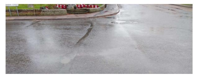
There are small areas that would benefit from the implementation of road markings and jointly, there are areas that would benefit from the removal of road markings. The introduction of edge of carriageway lines or the improvement to existing edge of carriageway lines would act as a means to reduce the perception of carriageway
