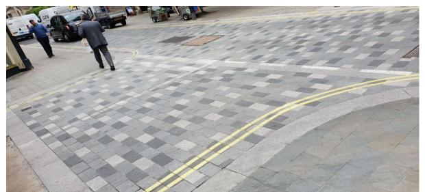
Figure 31 – Example of attractive raised junction with surface materials
